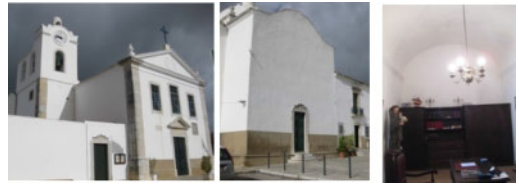
Figure 7. Lowered barrel vault in the church of Nossa Senhora do Carmo , in Fuzeta.
