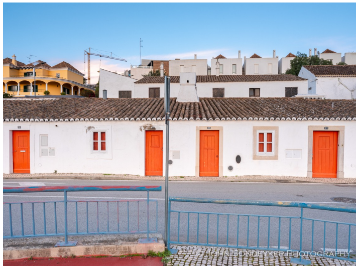
Colorful streetview with the housing project above.
