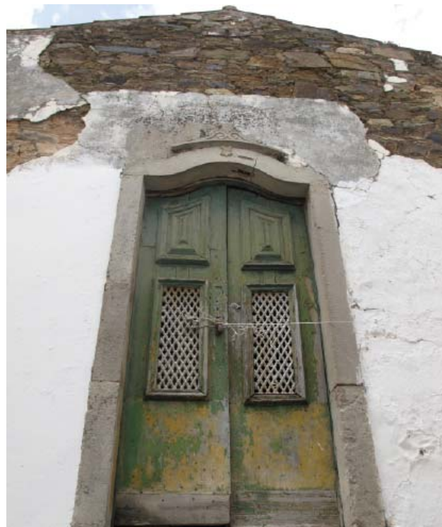
7] Shale stone wall of the Serra do Caldeirão coated with lime mortar (argamassa de cal). Doorway framed with expensive decorative limestone expressing the importance of the building or the wealth and social status of its inhabitants
