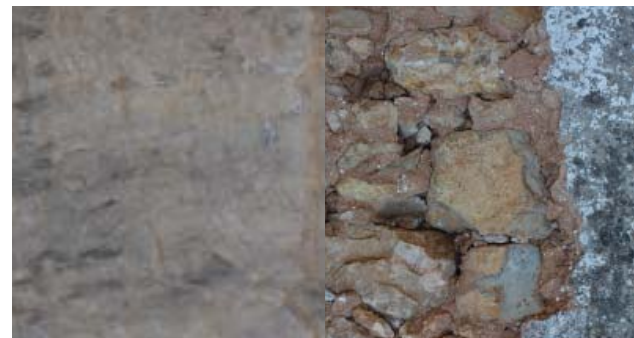
2] Strong limestone used predominately in stonework around the more affluent central Algarve (Alvenarias de calcário)
