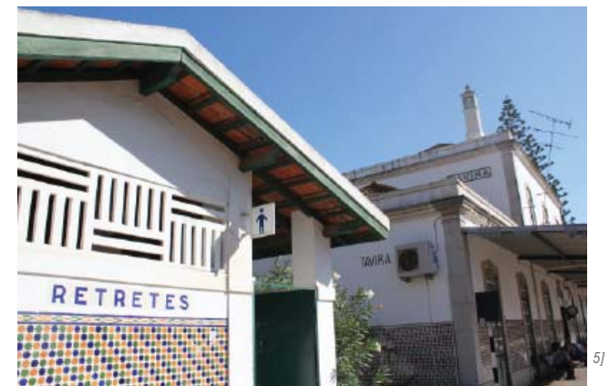
5] Regional Train station on the Algarve line, Inspired by Raul Lino's Casa Portuguesa (Portuguese House) style, homogenizing various different regional styles into a more "national" interpretation of Algarve architecture / Tavira
