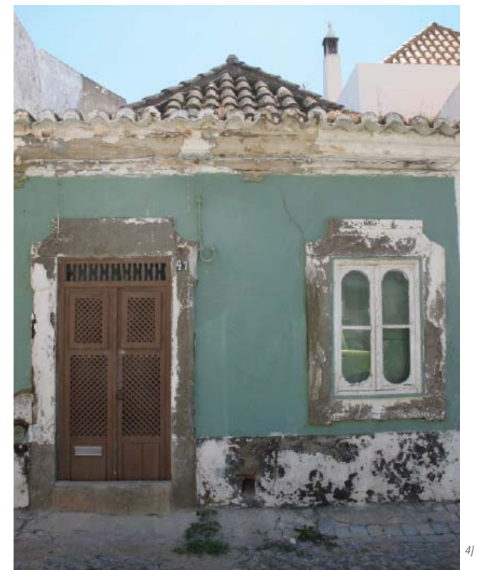
4] House in Tavira with the infamous four water tiled roof ( telhado de tesouro ), composite eaves ( beirado composto ) are also created by a series of different sizes of protruding terracotta clay tiles which are plastered in a way to form a decorative combination of undulating curves and ridges.
