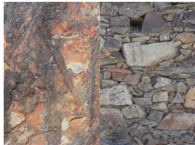
1] Shale rock of Serra do Caldeirão / Application in vernacular walls (Alvenarias de xisto azul)
