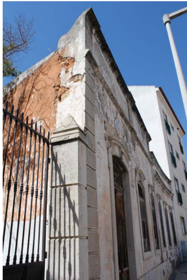
6] In the more affluent central Barrocal region, treatment of eaves became something of a symbol of social status. People began to use parapets (platibandas) as decorative features on the facade of buildings. Used to conceal the eaves along the facade. Acting as an assertive construction feature the parapet heightened the building giving it significant visual importance and expressing the wealth and status of its inhabitants. This photograph also shows the undecorated side of the build simple coated in clay mortar (argamassa de barro)
